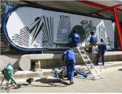
Sandblasted artworks on the glazed sections of the BRT station entrances. Source: www.onair.com
