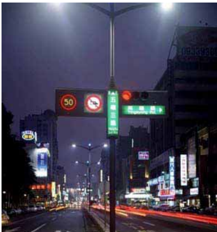
Utilization of solar power in Street Lighting, City of Kaohsiung. (Charles Lin)
