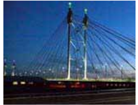
The Nelson Mandela Bridge, Newtown
